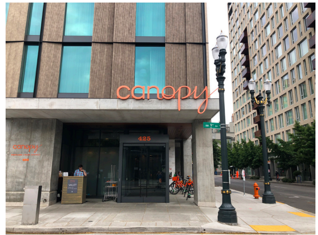
Channel lettering using printed Performance White on Black applied to translucent white acrylic. Sign appears colored in the day.
